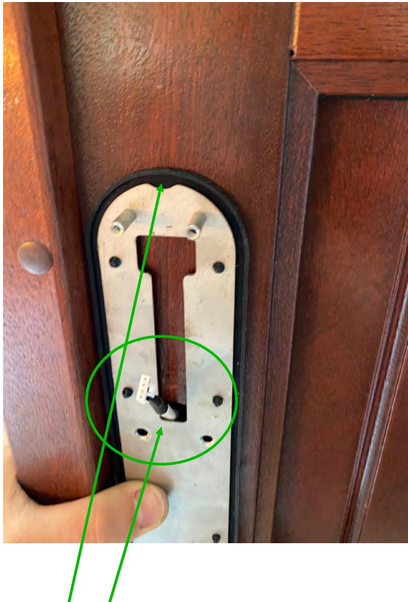
Use your hand to hold the front panel and the back mounting plate together.
