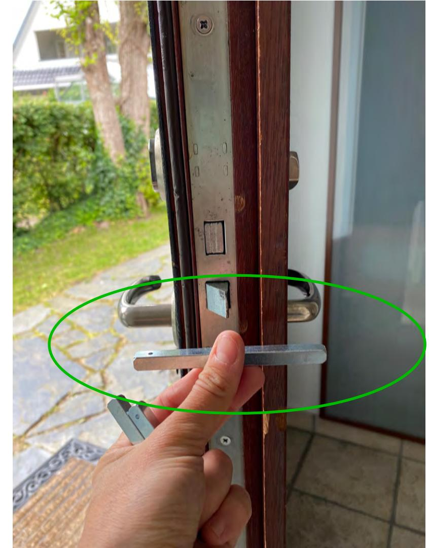
**XLOCK TIP:** This is a very important step! As this square shaft is the part that connects the front and back panel. Check page 23 for more detailed pictures of the installed square shaft.
