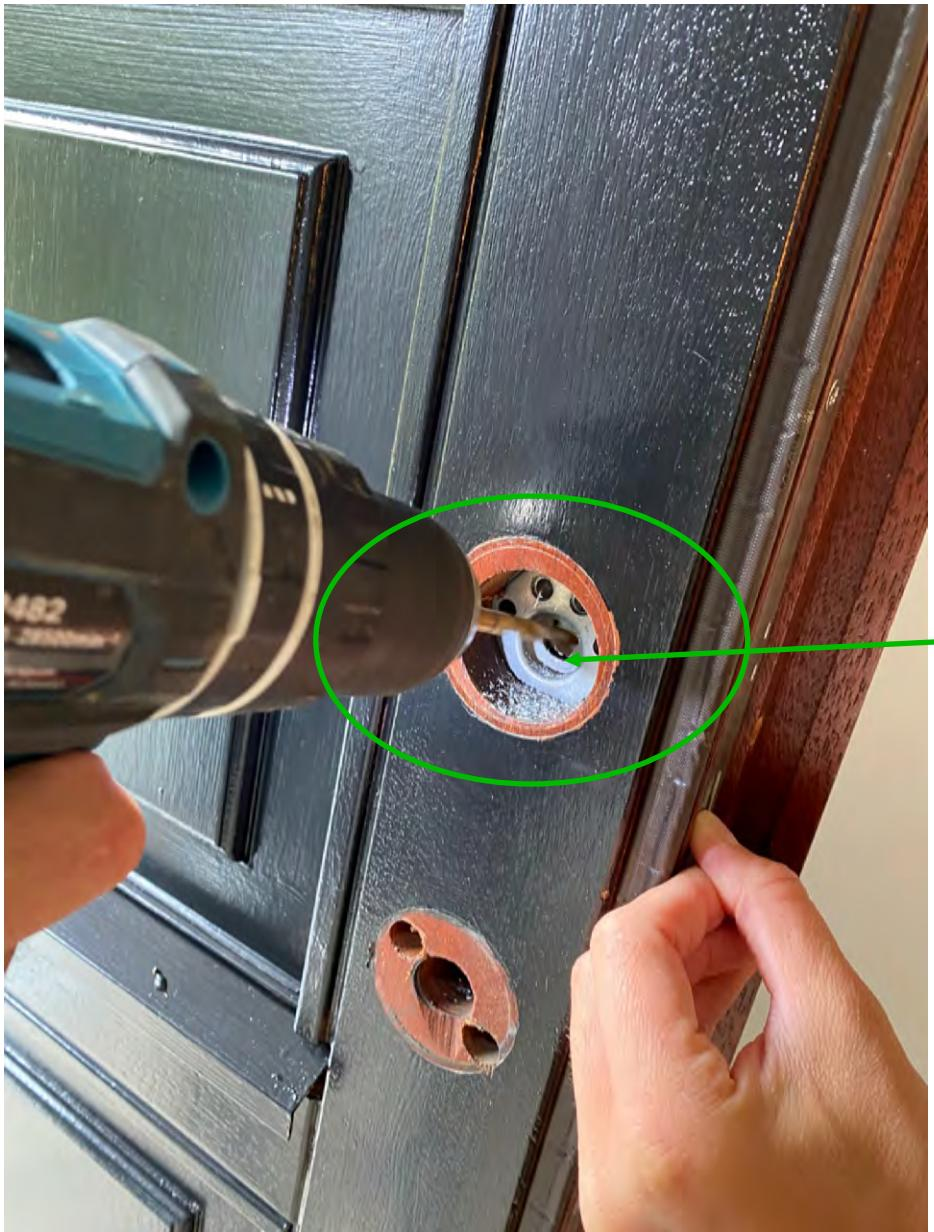
In some cases you might need to drill a bigger hole in the mortise lock to fit the cable through.
